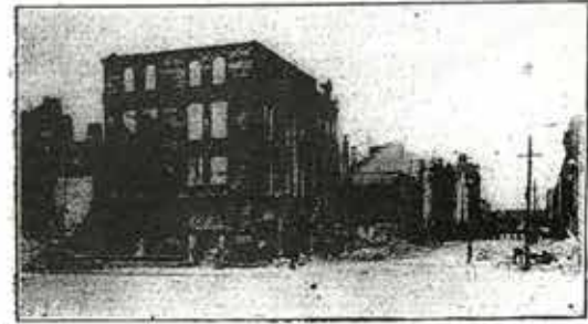
THE BOMBING REMAINS, LOWER PART, WERE DESTROYED, ONE OF THE REMAINS TO BE SEEN IN THE DISTANCE.
